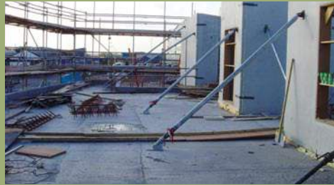
SOUTH WING PRE CAST UNITS
